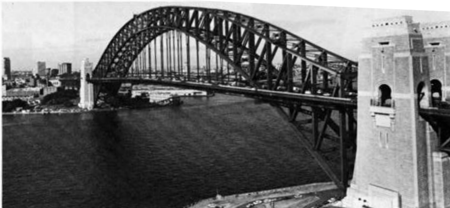
The 52 800 tonnes of steel in the Sydney Harbour Bridge are protected against corrosion by painting. Repainting is the full-time task of an engineer, three foremen and thirty maintenance workers. The cost of corrosion prevention is over $1 700 000 a year.
